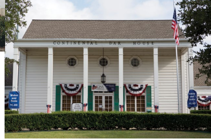
CONTINENTAL DAR HOUSE, DALLAS, TX
